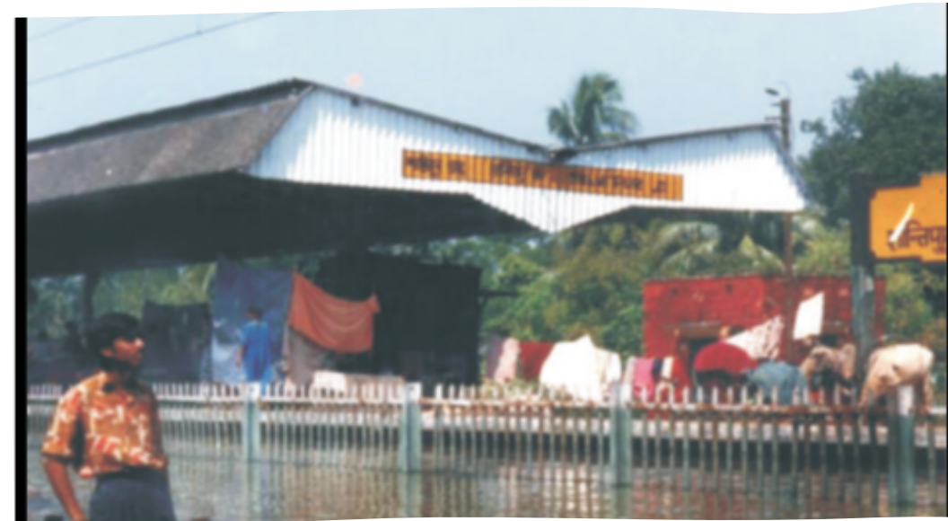
Flood Situation in Santipur Railway Station
