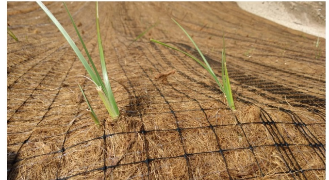
VETIVER Grass crossing erosion control blankets.
