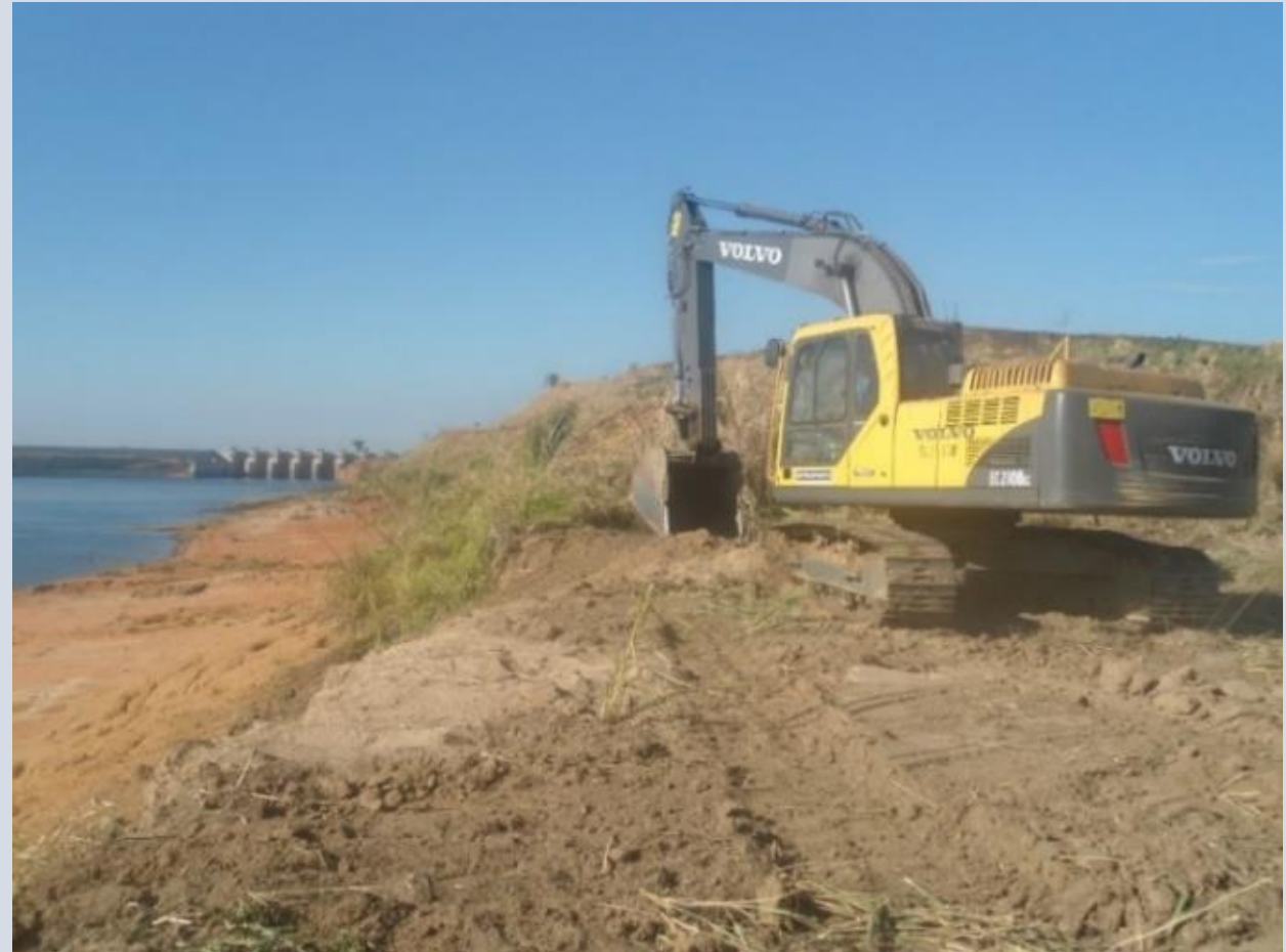
Site preparation for Vetiver planting
