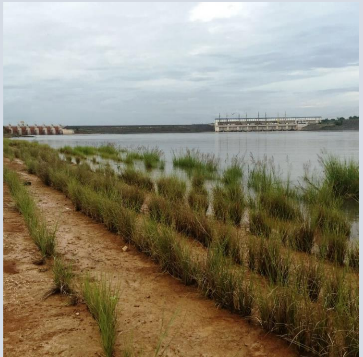
Vetiver was inundated after heavy rain overflow
