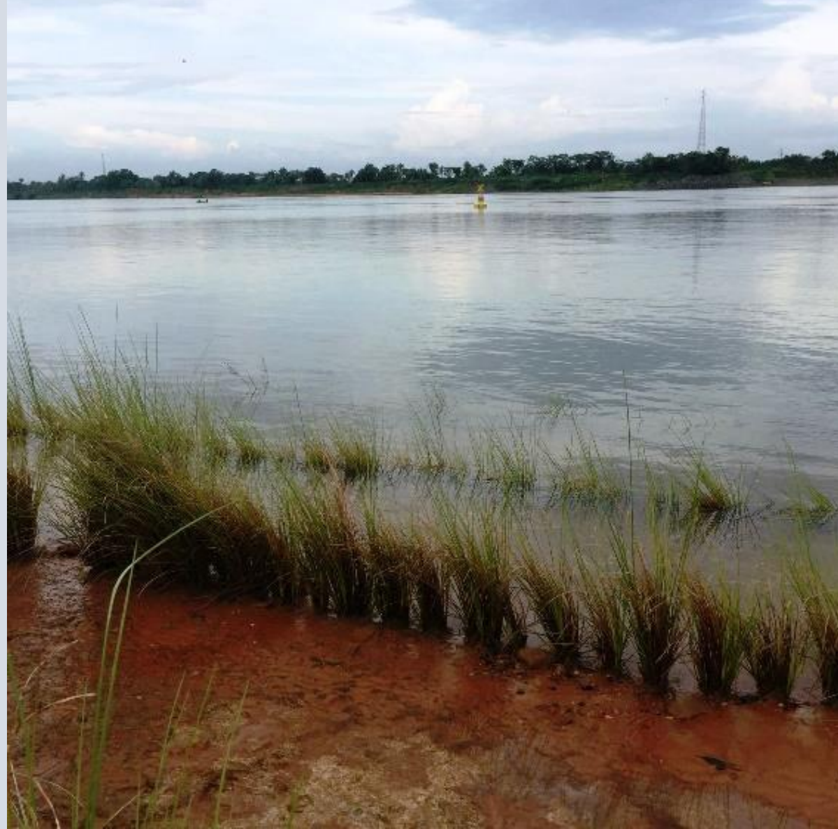
Vetiver was inundated after heavy rain overflow
