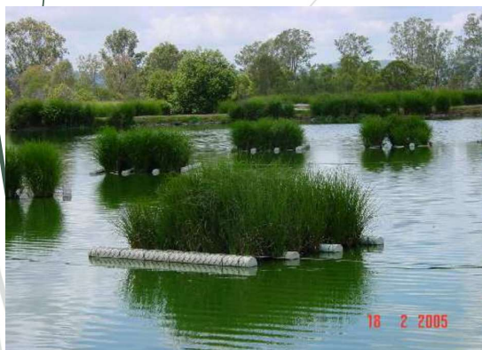
Floating treatment platform (FTP)
